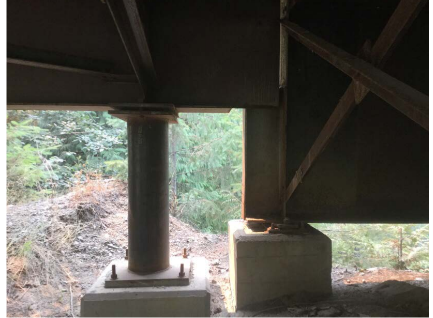
Right bank piers, separate for each span
