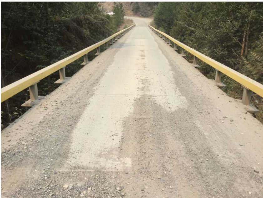
Right bank jump span deck
