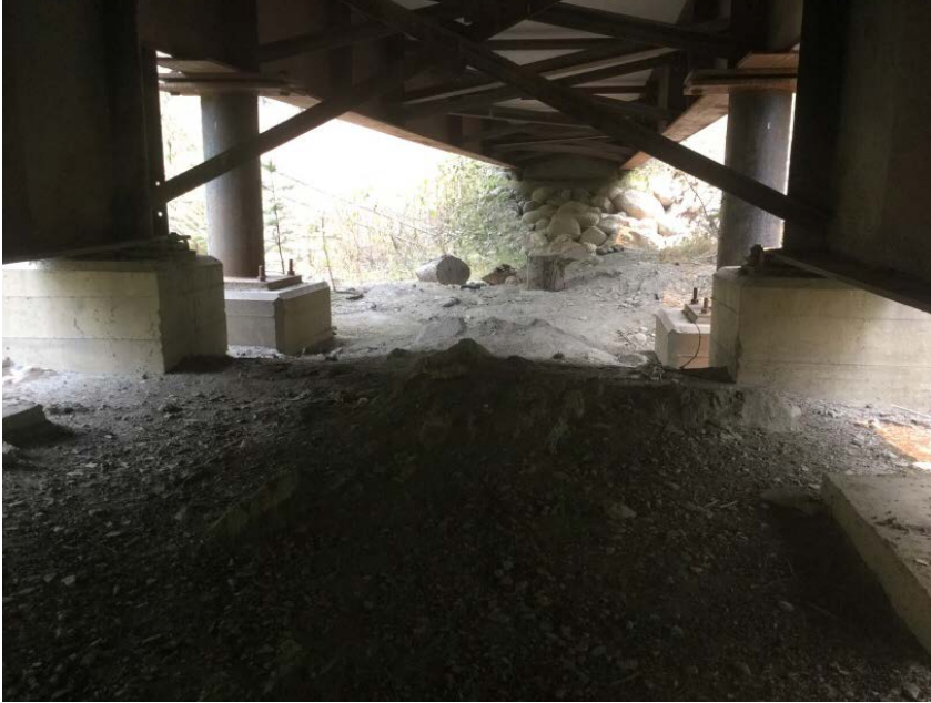
Main span right bank abutment
