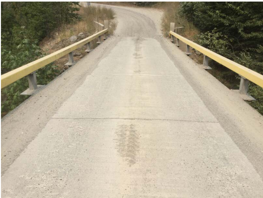
Left bank jump span deck
