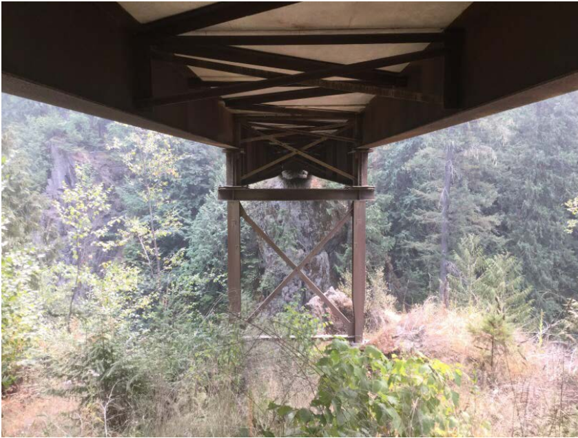
Left bank jump span superstructure and left bank bent
