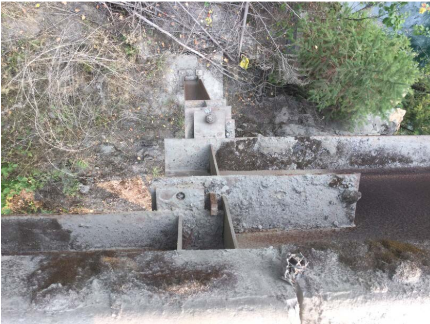
Welded restrainers for left bank jump span
