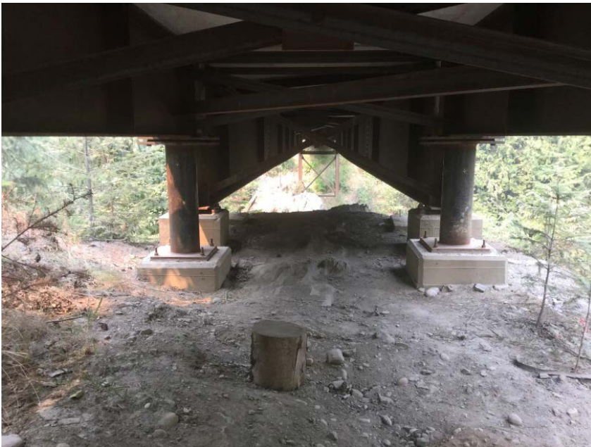
Right bank jump span pier, with main span pier behind
