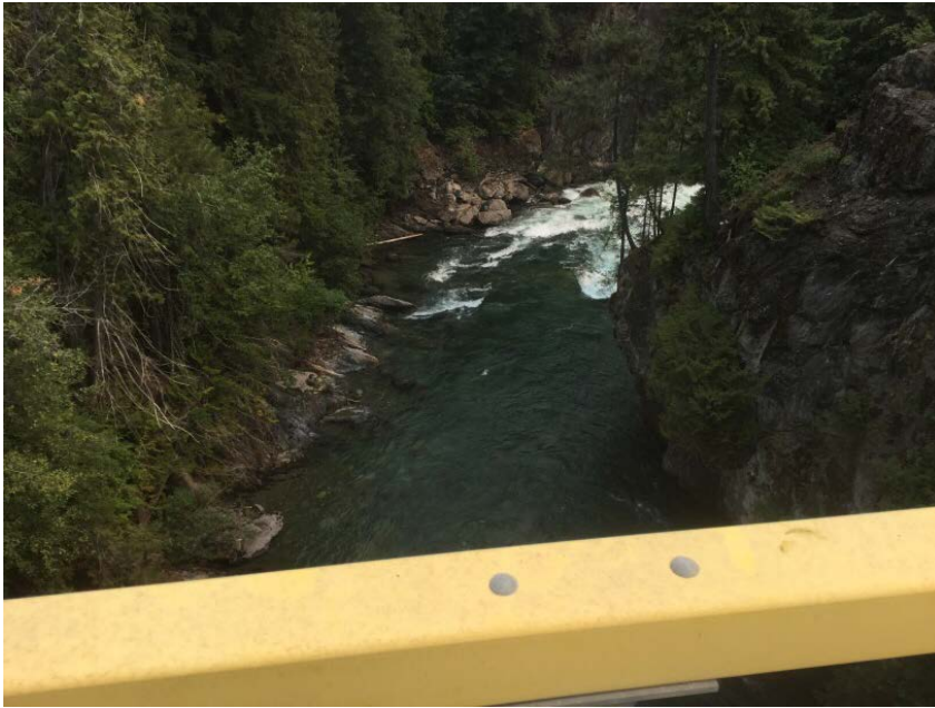
Looking downstream from deck
