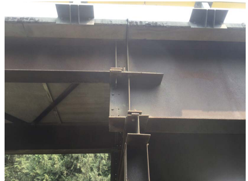
Left bank jump span to main span connection
