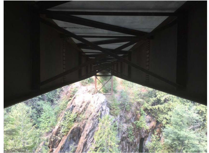
Main span superstructure
