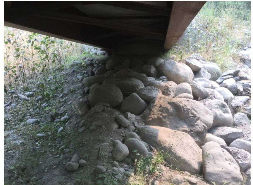
Right Bank Abutment when facing downstream
